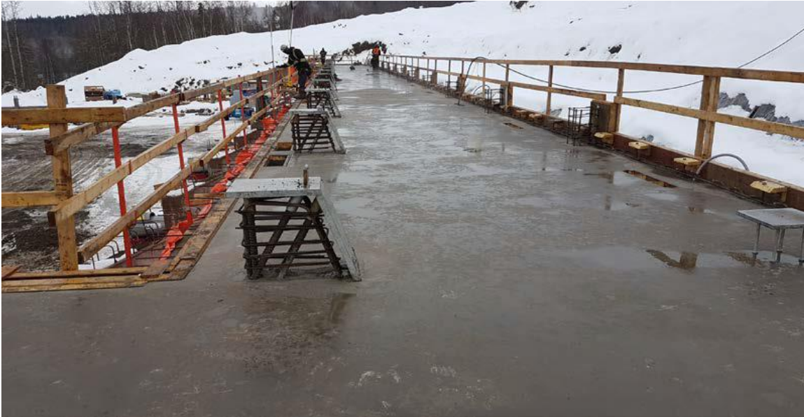
Portion of Concourse Slab is poured and finished.
