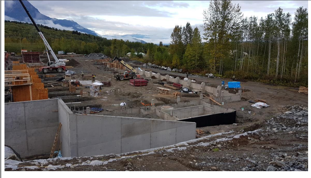
View from arena end looking towards ongoing footing preparations
